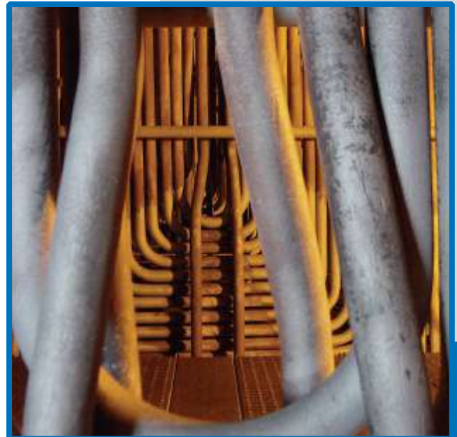
Unusually clean tubes, results occurred after use of the TIFI program for a 5-month period
