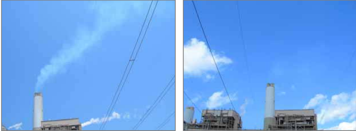
Figure 5 No Visible Opacity issues with TIFI treatment on the right photo with both stack inlets at an SO 2 concentration of 2.9#/10 6 BTU
