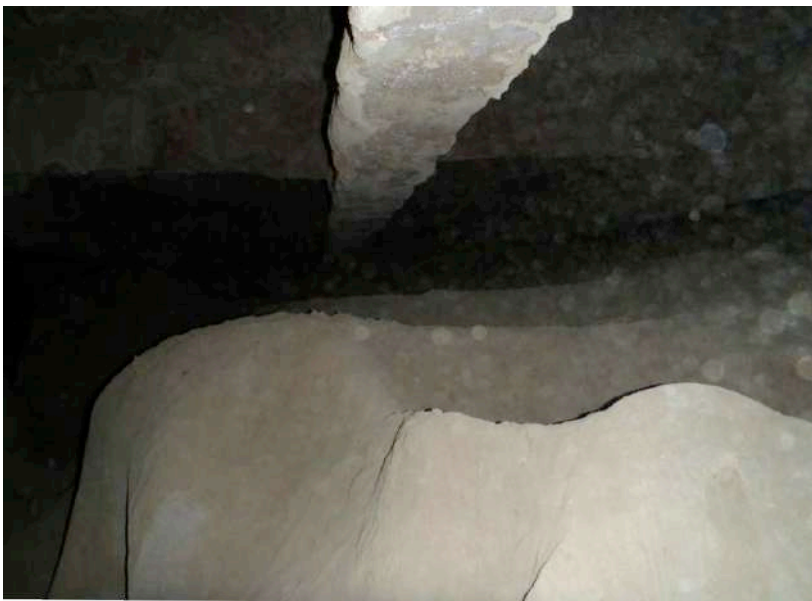
Figure 1b: South Side A SCR, Layer 2, 2 nd Catalyst Module Seal Strip
