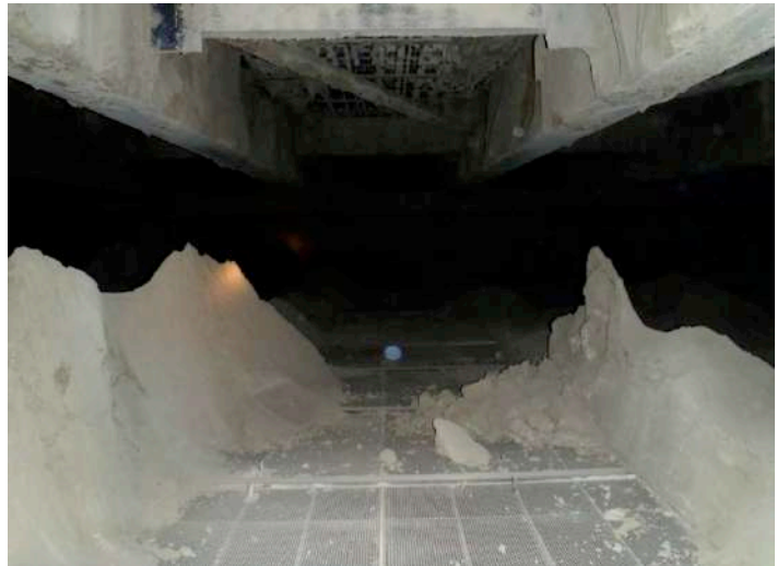
Figure 12a: Beam ash slough (left)
