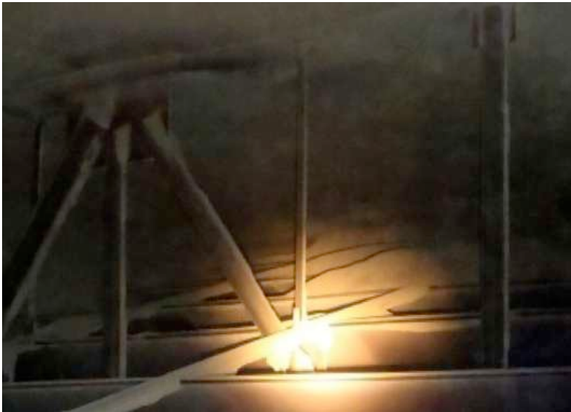
Figure 1a: Flyash on Turning Vanes
