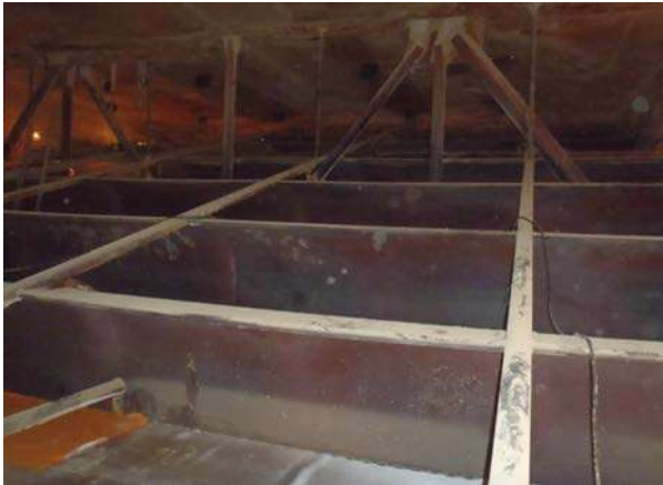
Figure 5: Turning Vanes & Center Truss
