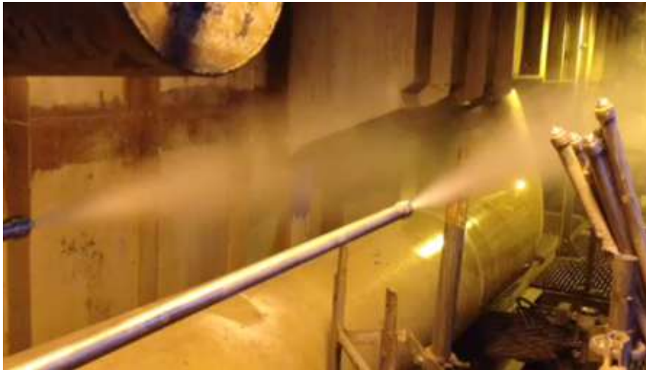
Figure 7. Air-atomized chemical injectors selected to produce droplet size distributions that rapidly evaporate water droplets, while delivering chemical to problem areas. Note the fine mist and absence of large, falling droplets.
