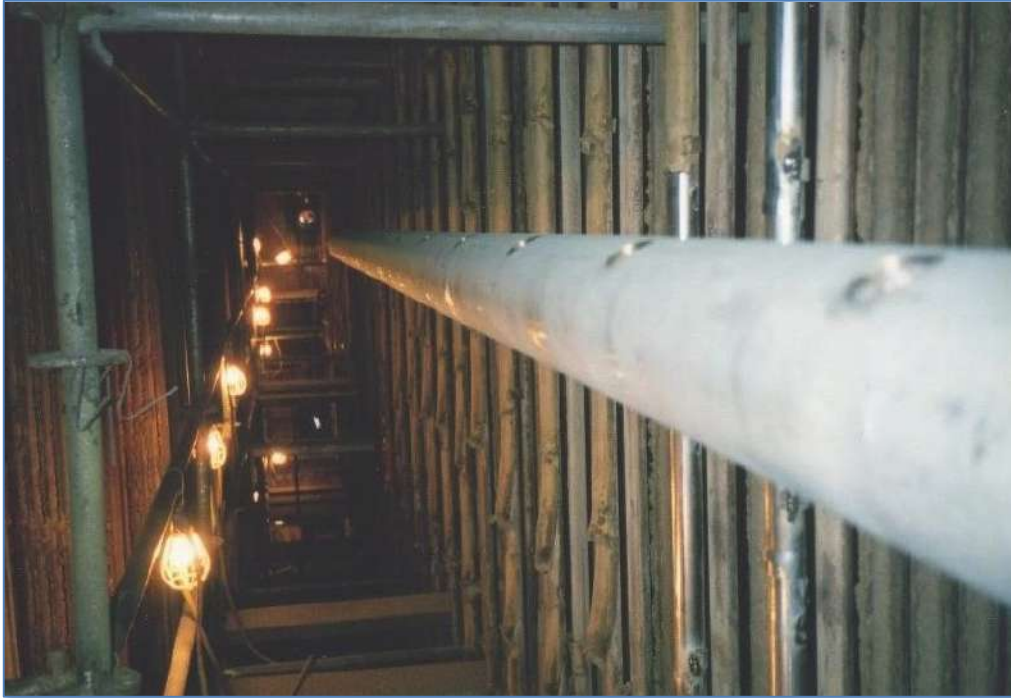
Figure 3 Multiple Nozzle Lance (MNL) injector is used for convective pass SNCR injection
