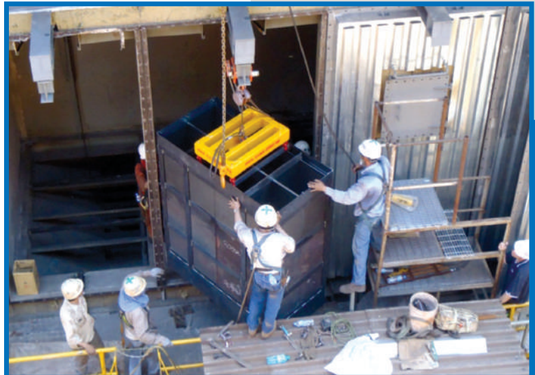
Catalyst installation
