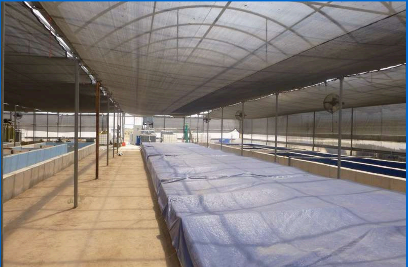
Figure 3: Concrete raceway covered during operation
