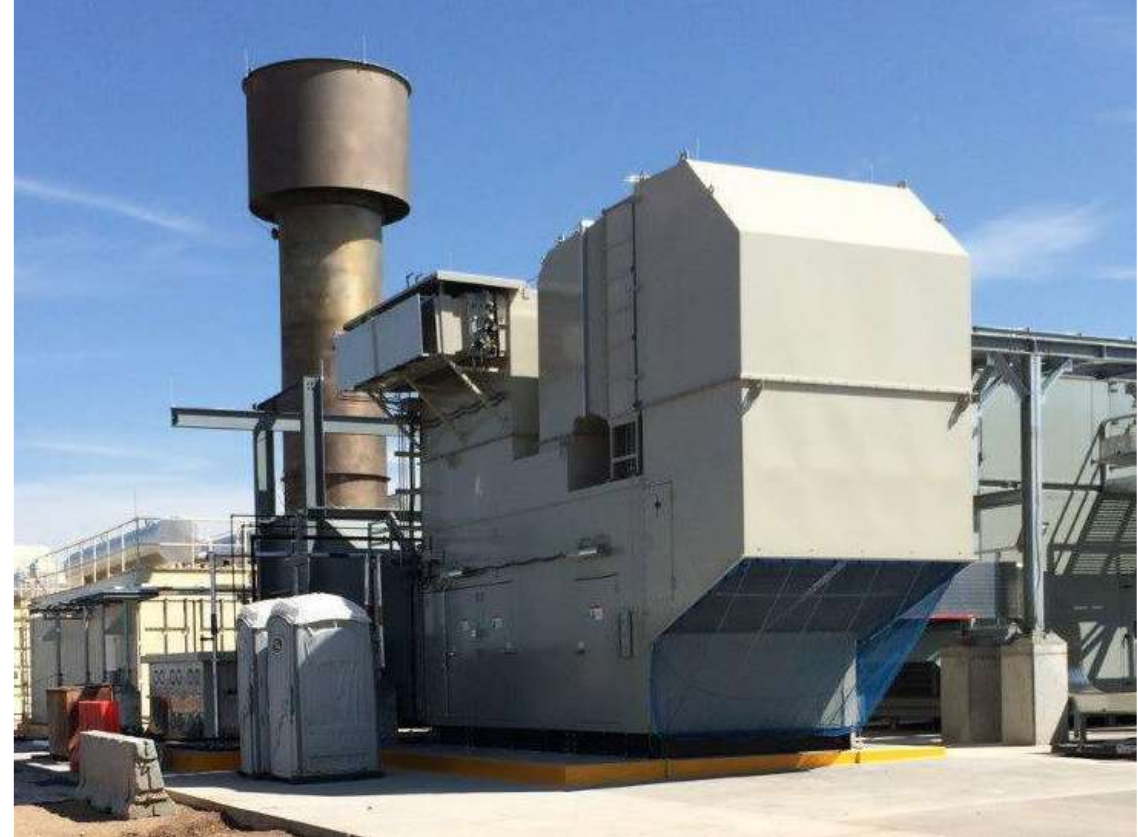
Fuel Tech SCR System with UDI™ Urea Direct Injection
